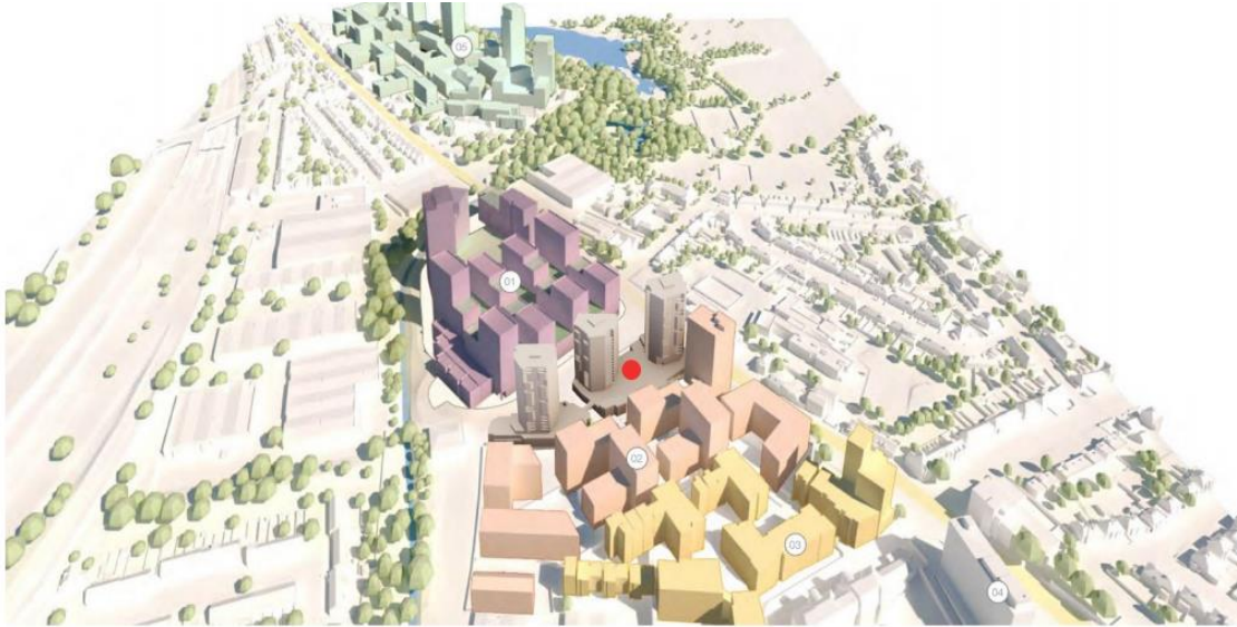
(image looking from NE to SW)
